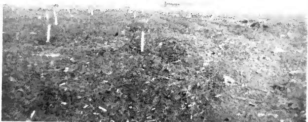
A cleared and graded peat bog, ready to be planted over to cranberry vines.
